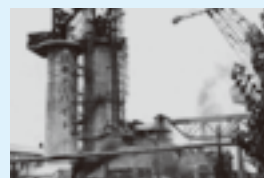
Handling system for a chemical fertilizer plant (bucket elevator)
