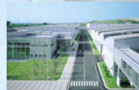
Kyotanabe Plant, the mother plant for chains
